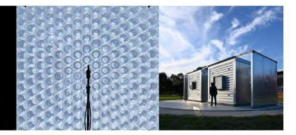
Under" roof. The roof hovers above the space and lacks detail, acting as a horizontal screen, stretching towards the microclimates at either end. The roof allows rainwater to flow from one end to the other, where it is collected and directed with rain chains to the wild bamboo below. The rain becomes an auditory spectacle made available through a small window in the northern wall.
